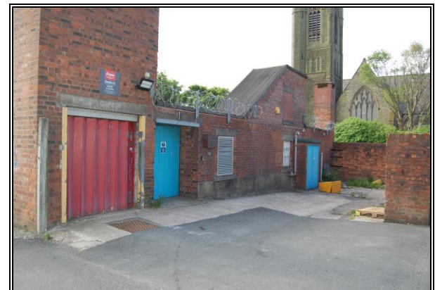
Rear Delivery Bay
